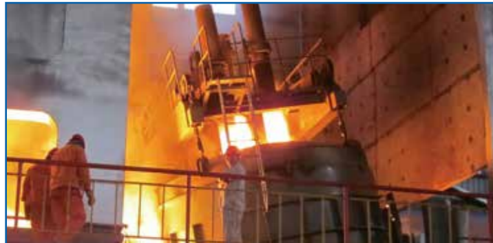
Electric arc furnace
